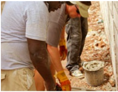
(The work team building onto the school)
