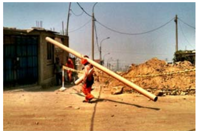
(Construction worker installing water pipes.)
