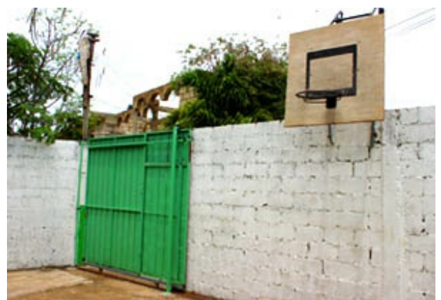
(High walls and iron gates to prevent unwelcome visitors.)
