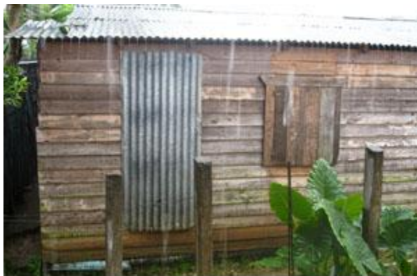
(Typical wooden house with sheet metal. It's raining hard.)
