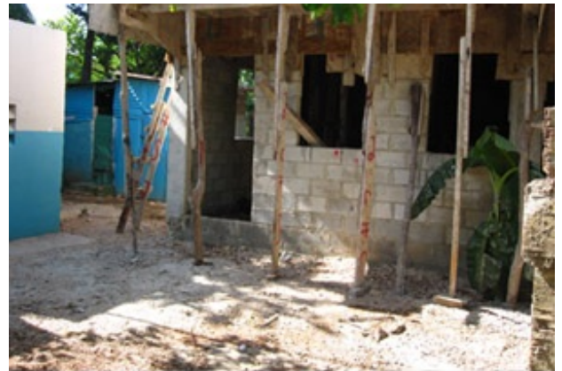
(Construction of 3 new classrooms.)
